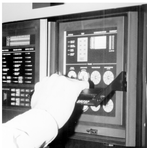
Press latch and pull to disengage handle
